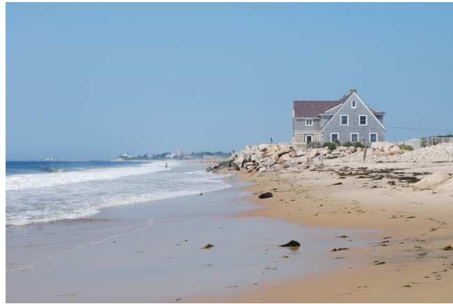
Figure 9.3: Beaches houses on the western side of Misquamicut Beach, Westerly, Rhode Island.
