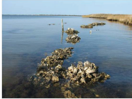
Figure 9.2: Artificial oyster reefs parallel to the shoreline provide a way to slow the rate of coastal erosion by reducing incoming wave energy.
